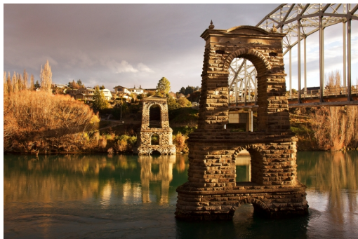
Alexandra_Bridge_Piers Merit Graham Phillips
